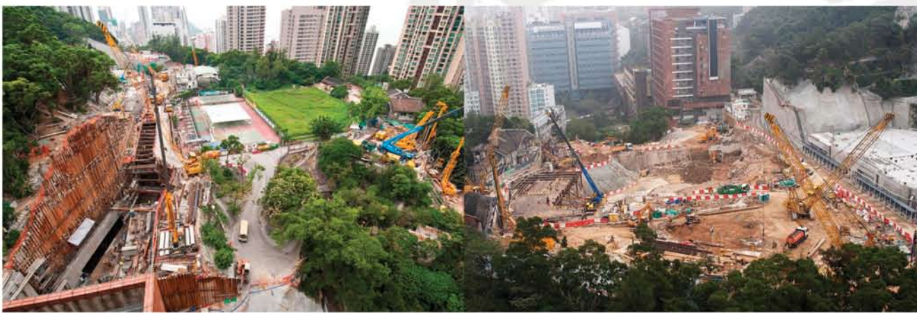
Centennial Campus under construction July 2009, March 2010
