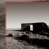
The school house in Qunu was a single room with a tin roof. It stood on the other side of the hill from the village. Mandela remembered his first 'school uniform'.
